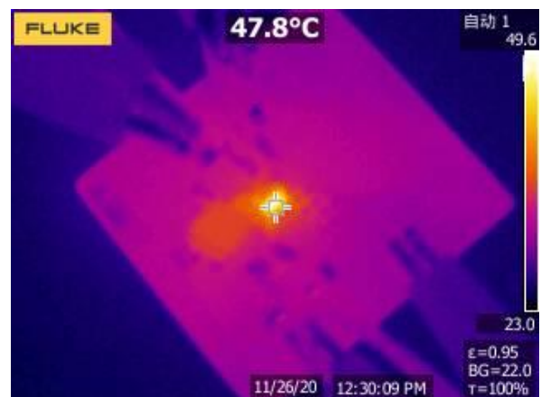
Figure 23. Thermal, 24VIN, 5Vout, 0.6A
